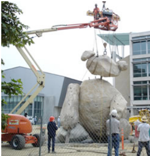
Artist Tim Hawkinson (lower left) and construction crew position the head on his giant rock bear. Behind 'Bear' are the Calit2 Building (left) and the Computer Science and Engineering Building, both under construction.
